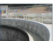
Following long term difficulties with scraper bridge operation being disrupted by degradation of concrete forming the outer tank wall, and a solution involving mechanically fixed steel plates not having provided a long term fix, Ram Services Limited developed a solution to permanently repair the tank walls and maintain the operation of the scraper bridge.
